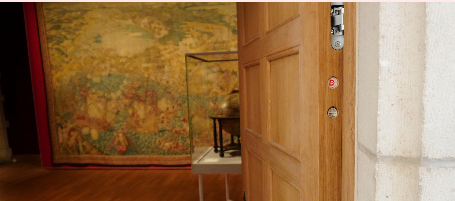
Brandwerende deur in Museum Hof van Busleyden, Mechelen © BWZR
